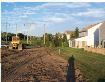
Restoring residential area
