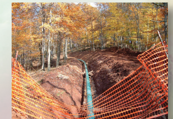
Pipeline in trench
